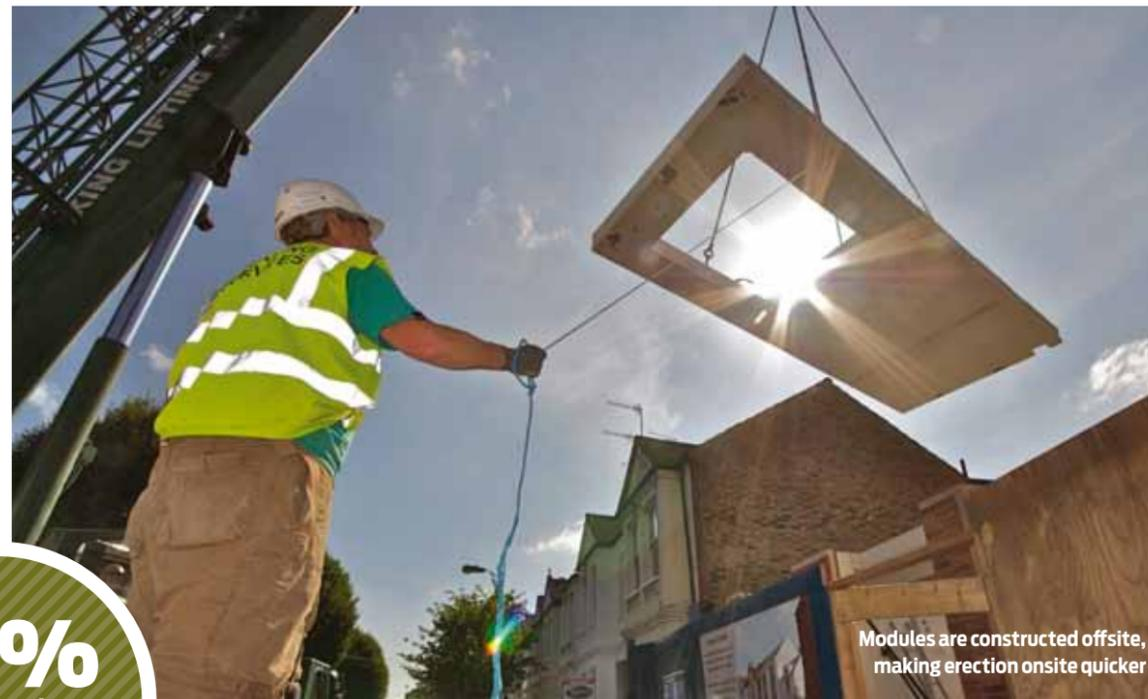
Modules are constructed offsite, making erection onsite quicker
