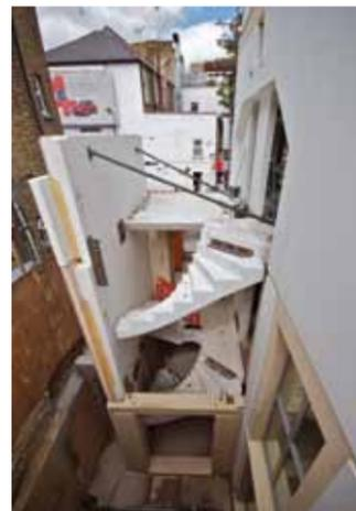
The helical staircase provides natural stack ventilation
